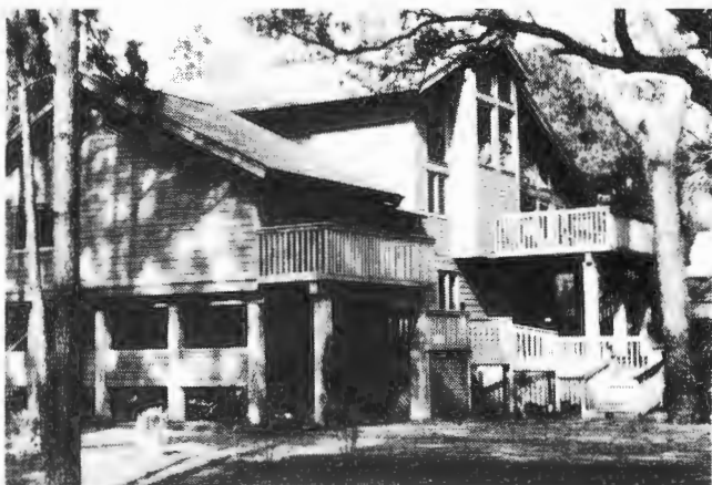
Figure 4.3. Elevation by Posts
