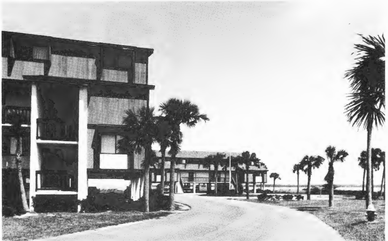
Figure 3.34. This structure uses a mixture of materials, texture and color very successfully and provides a variety of form for visual appeal. The space under the building remains open and light through a combination of white unobstructed walls and piers, landscaping, and layout relative to other buildings. A human scale is accomplished by breaking the building up into different heights and sections, rather than an imposing three-story box, as is often done (see also Figures 3.58 through 3.62).
