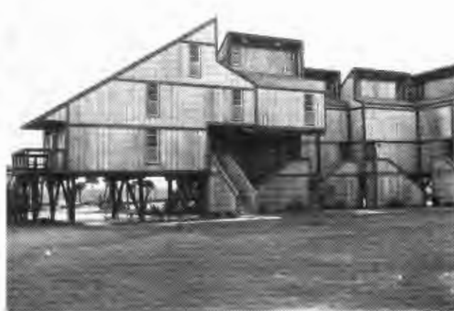
Figure 4.4. Elevation by Posts
